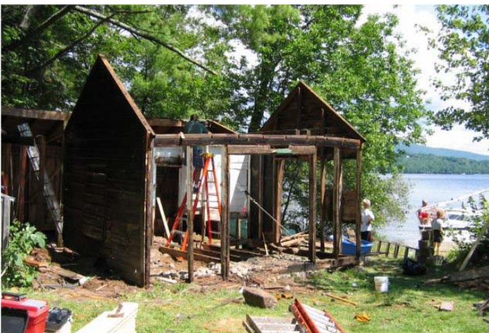
2) August 6, 2004: Starting to tear down the old Boathouse.
