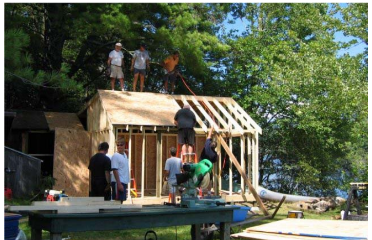
3) August 8, 2004: Putting together the new Boathouse.
