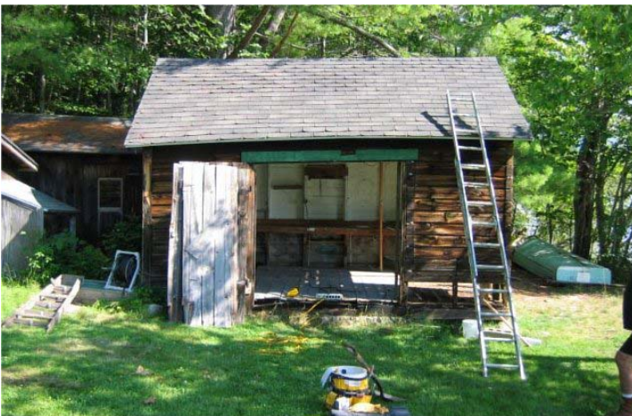
1) August 4, 2004: Getting ready to tear down the original Boathouse
